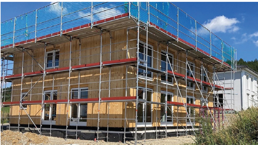
Advantages of MHM walls include short construction times and dry construction
