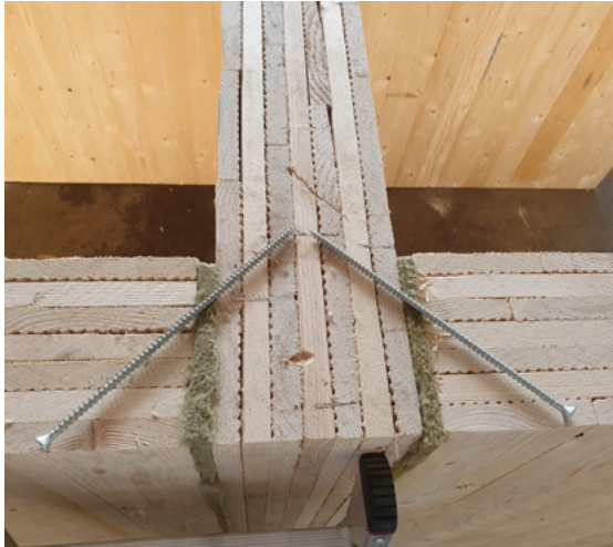
The MHM system offers sophisticated and tested solutions for fire protection and sound insulation
