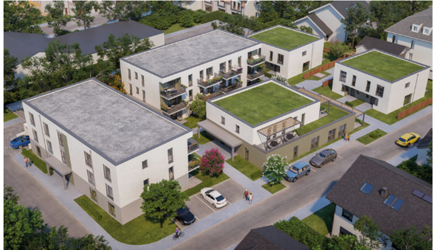
An innovative quarter in Berkheim designed by Wild Projektentwicklung: Part of the residential buildings also have MHM walls
